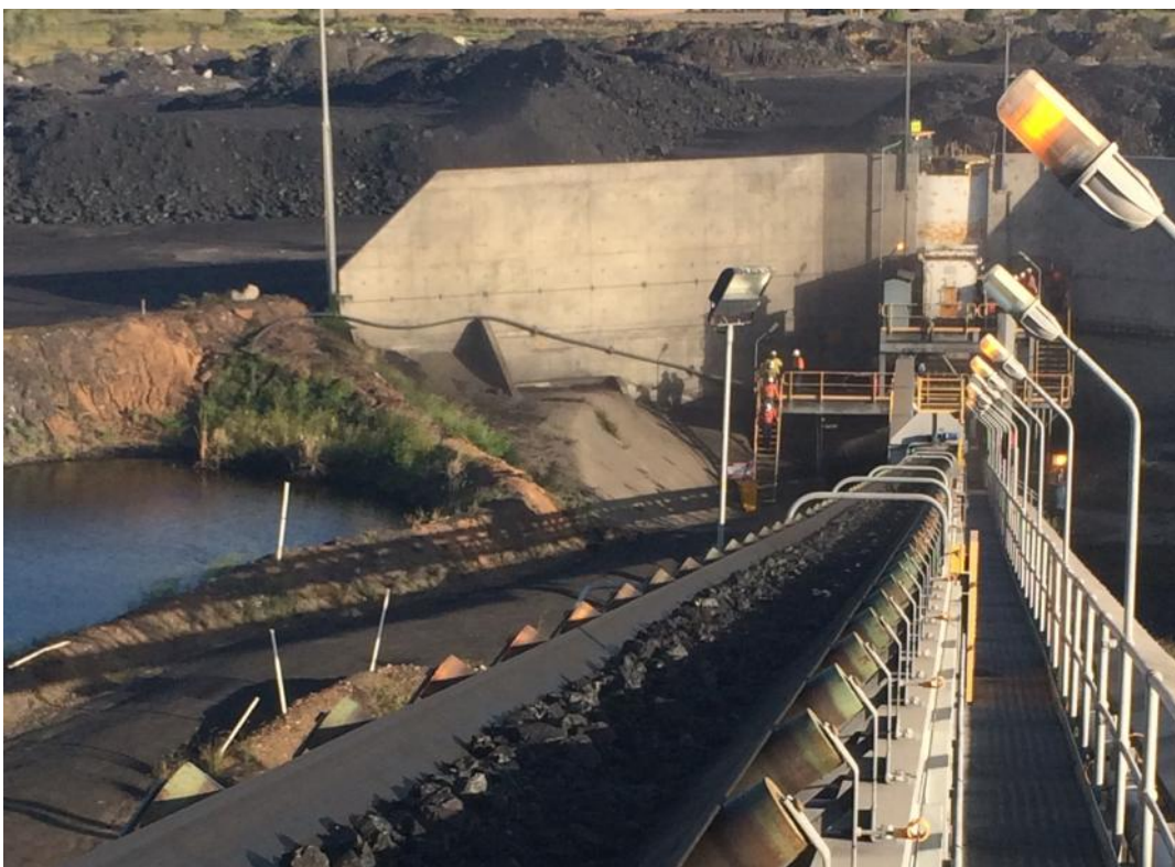
Image 2: Run-of-mine coal on feed conveyor
