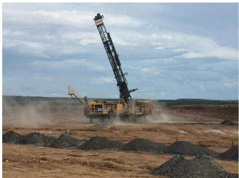
Production drilling in preparation for first blast
