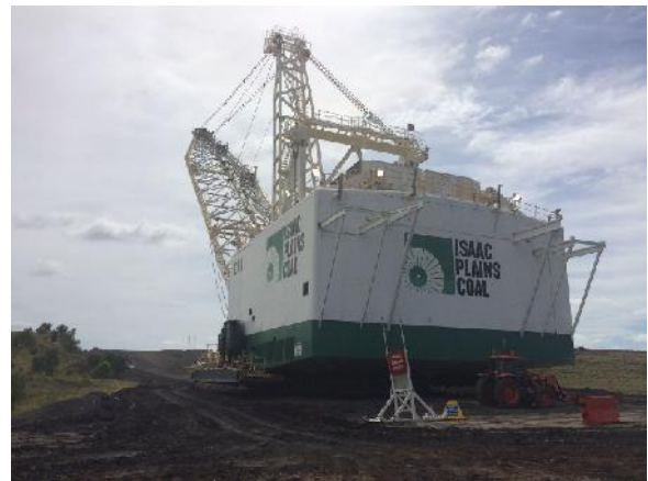
Dragline ready for operation
