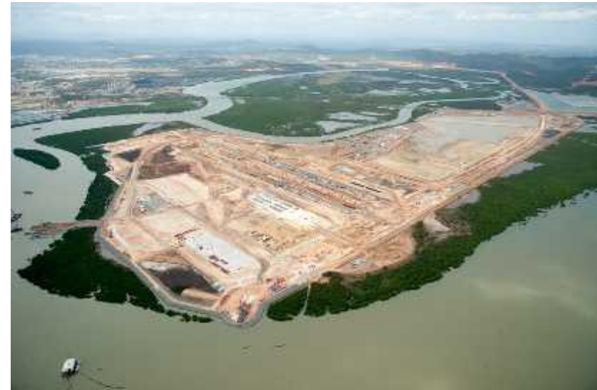
QLD port under construction – Wiggins Island
