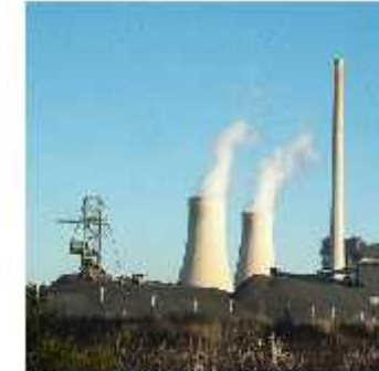
Bayswater Power Station.
